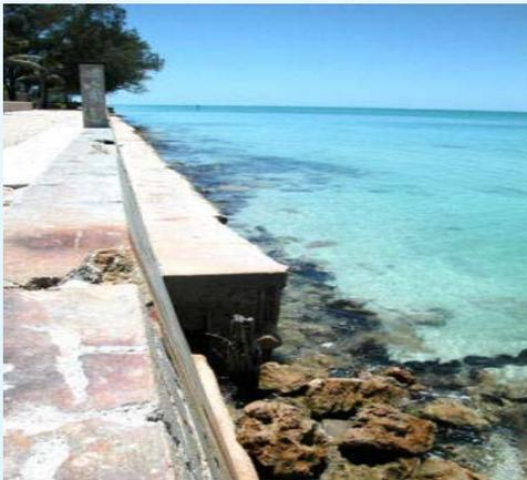
**Iguana burrows are common along seawalls on Gasparilla Island and their undermining may facilitate breaches during severe storms, especially hurricanes.**
