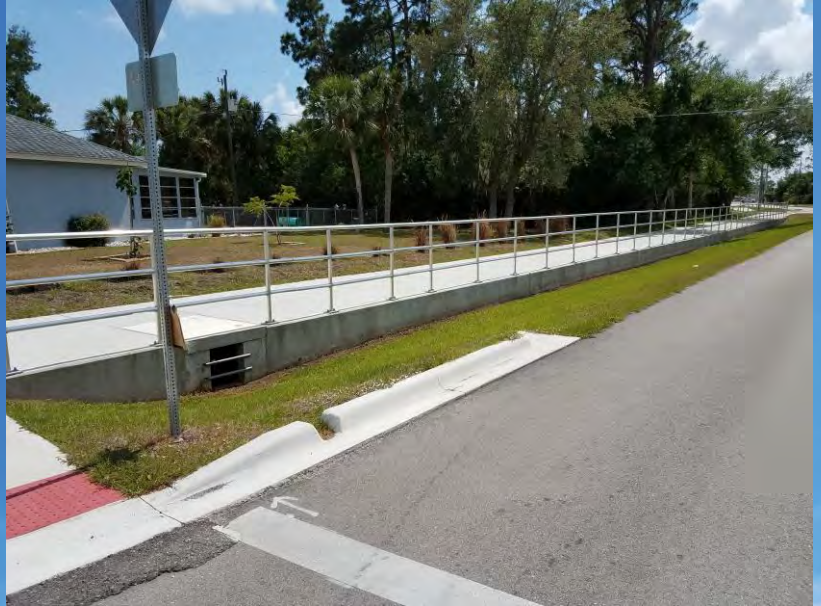
New pathway and drainage at West Tarpon
