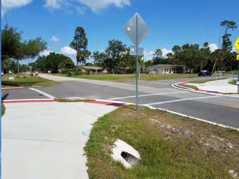
New curb, drainage, and pathways at Ambrose/West Tarpon
